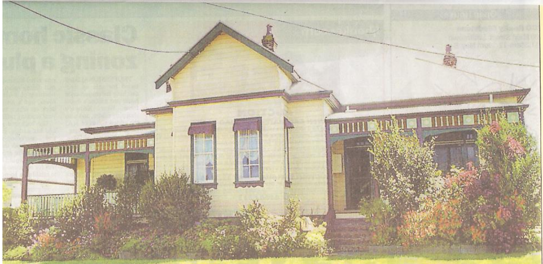
Watson House, built in 1885 (restored in 2004) (Photo Macleay Argus)
