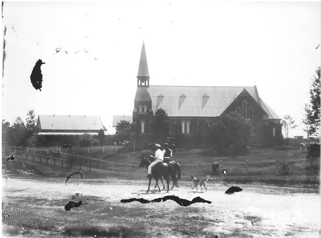
Church photo taken from southern side (Sea Street)
